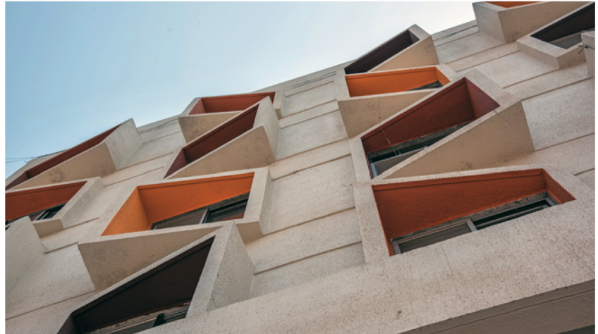
Nilaya project: The chajjas and sun-breakers were designed in a diagonal position so that the neighbouring buildings don't look into each other.
