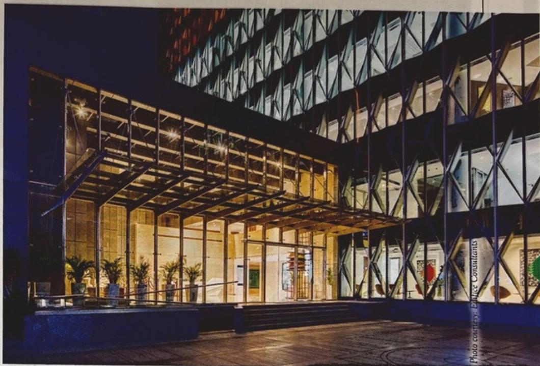
Supportive materials like jaalis , fins and screens help shield glass.
