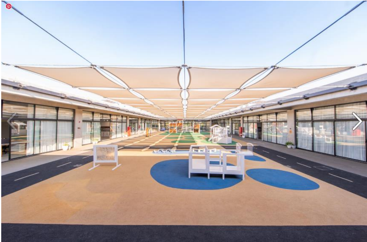
A large courtyard is at the heart of the project, guiding the layout and circulation within the school design Image: Courtesy of Heartfulness International School
